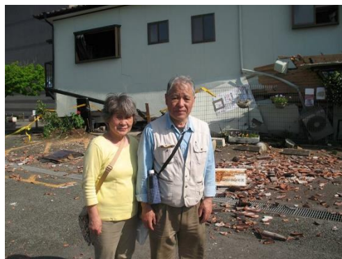
A pastor and his wife in front of a collapsed church
